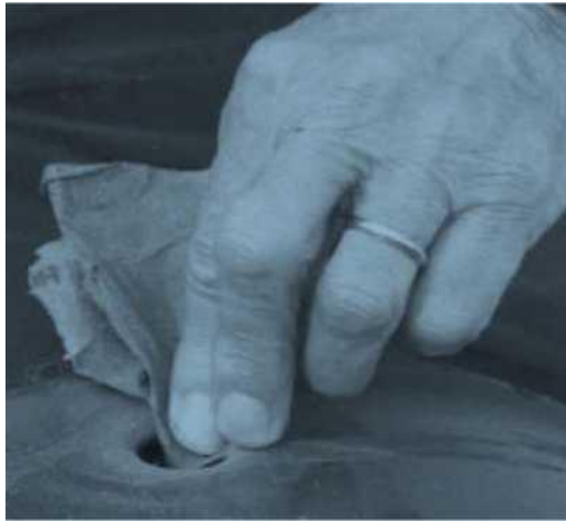
Thoroughly clean the pipe and driven-in hole with sand-paper
