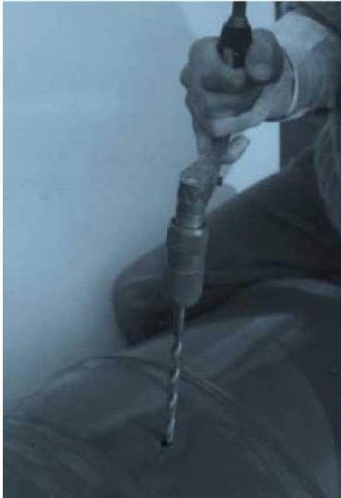
First, drill a hole of 6 mm and afterwards a hole of 16 mm into the marked spots
